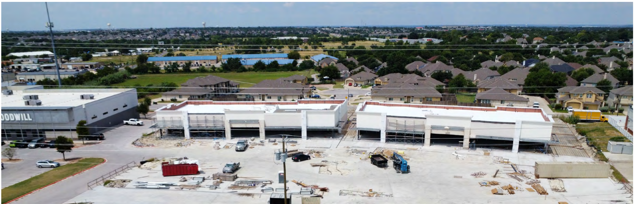
Construction Progression August 2025
