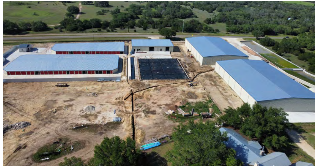
Construction Progression May 2025
