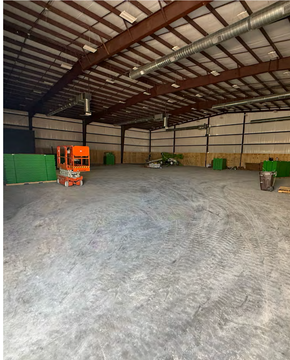
Construction Progression May 2025
