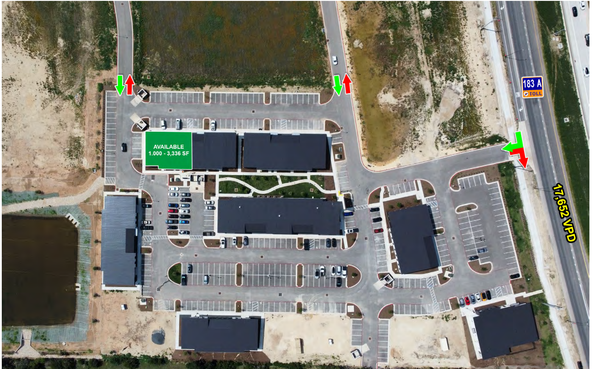
Construction Progression May 2025
