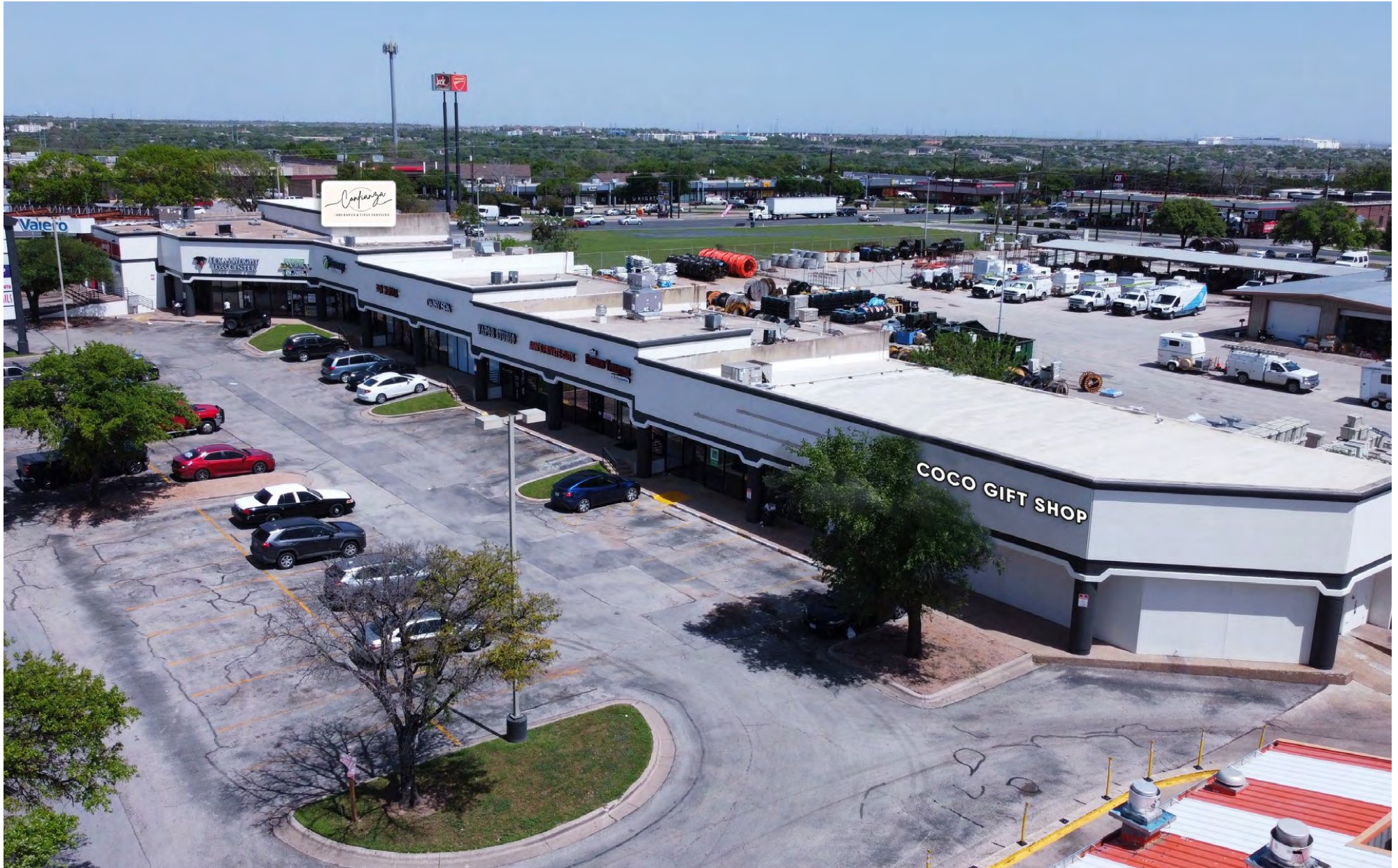
New Paint as of March 2024
