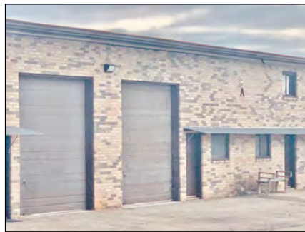
Dock High Doors C7 & C8
