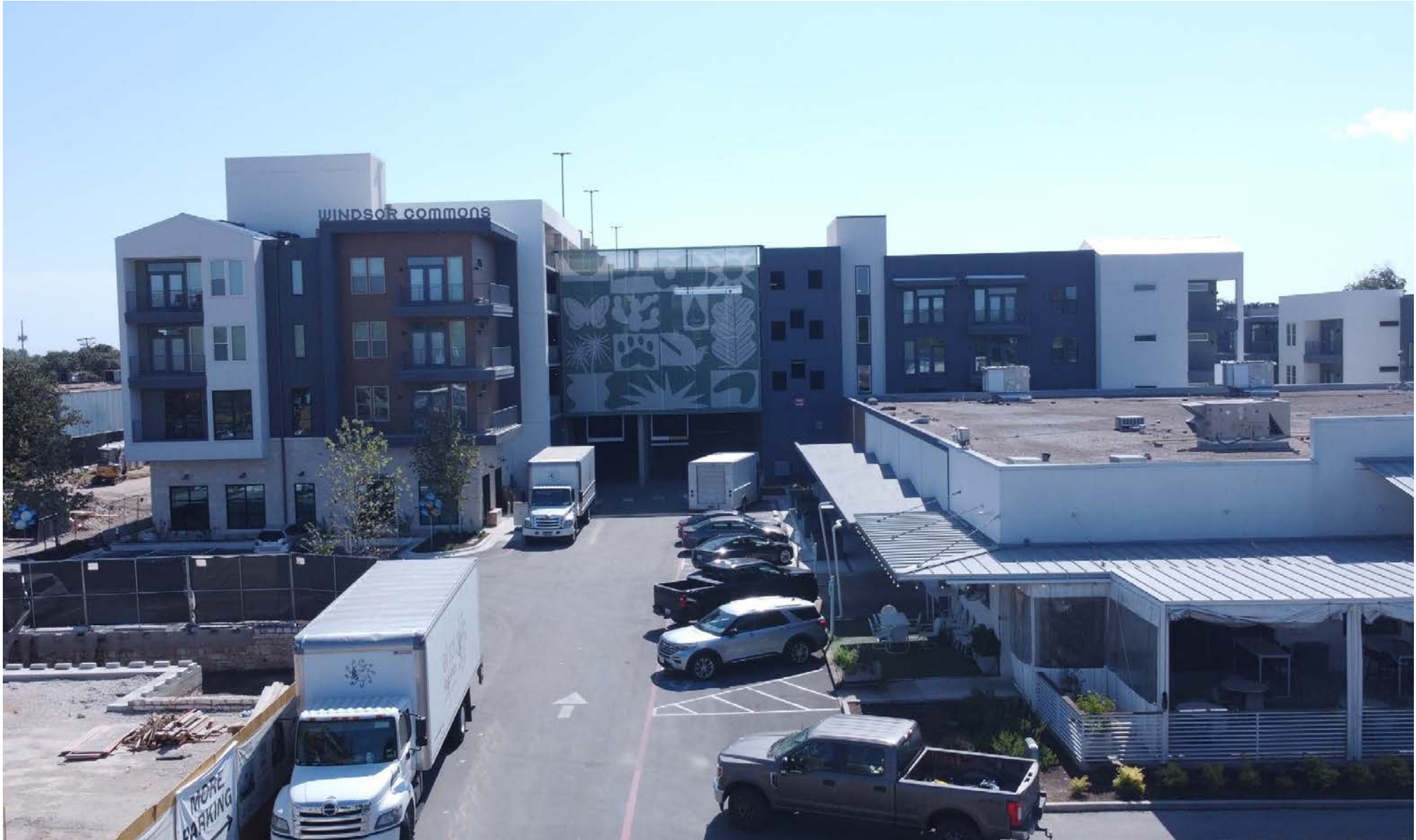
Construction Progression Sep 2024
