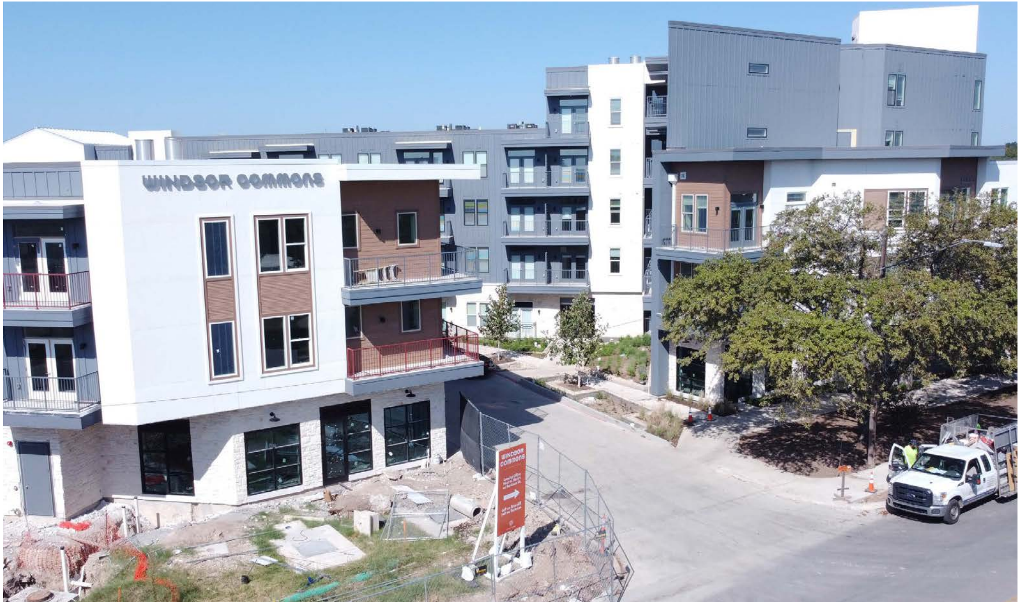
Construction Progression Sep 2024
