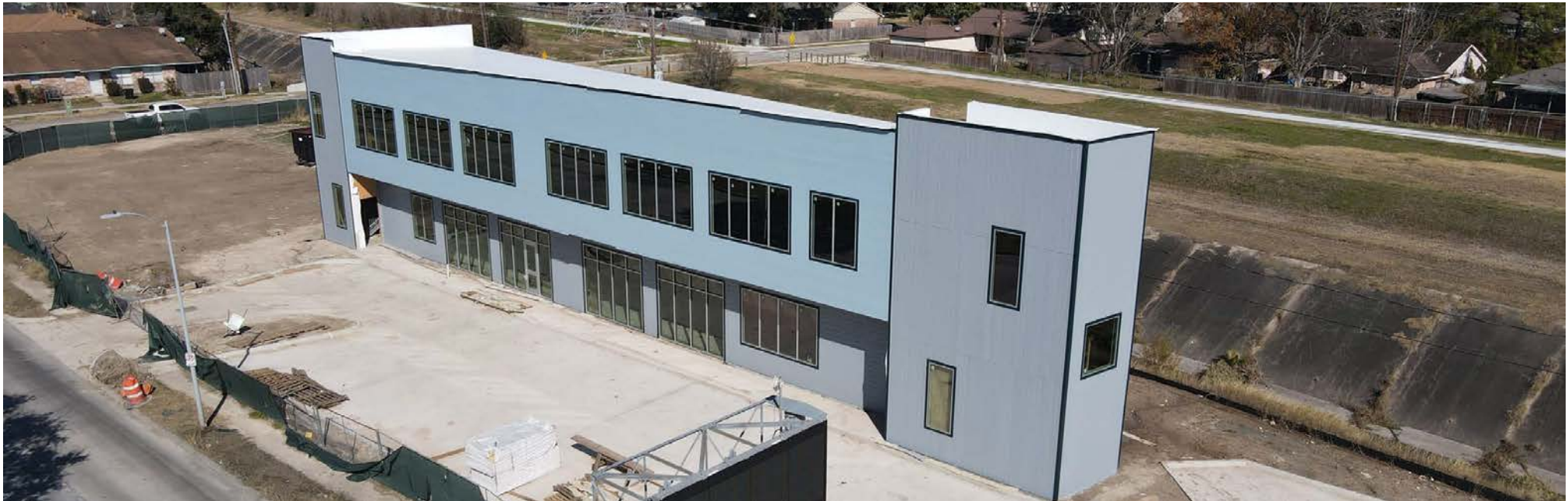
Construction Progress Feb 2025
