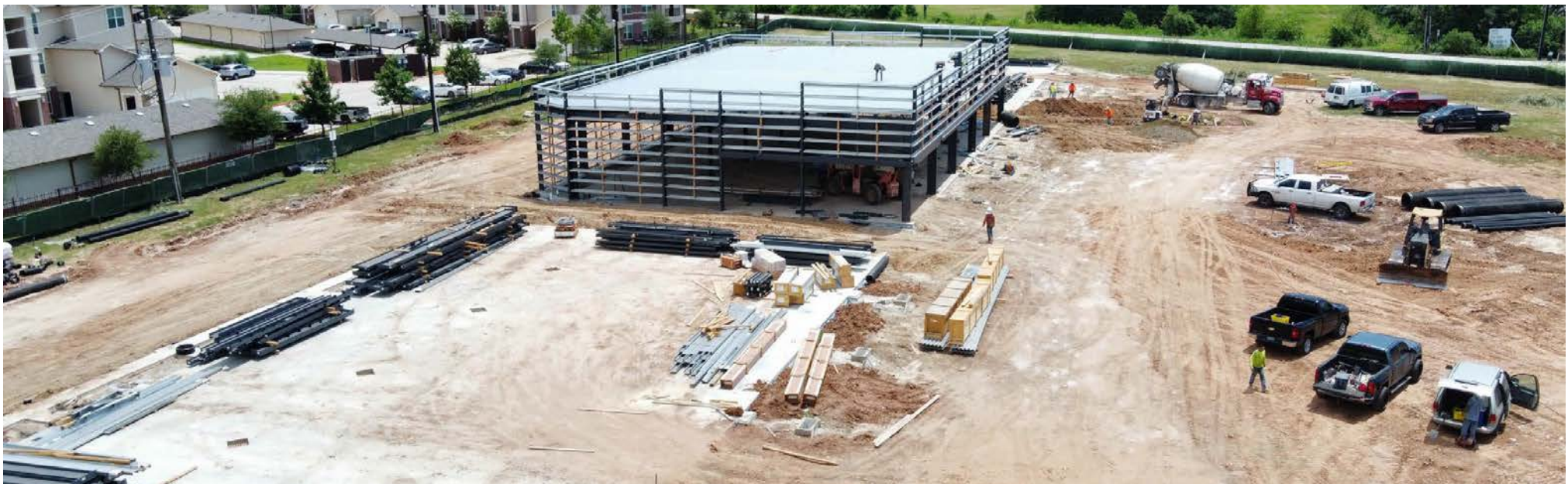
Construction Progression August 2024
