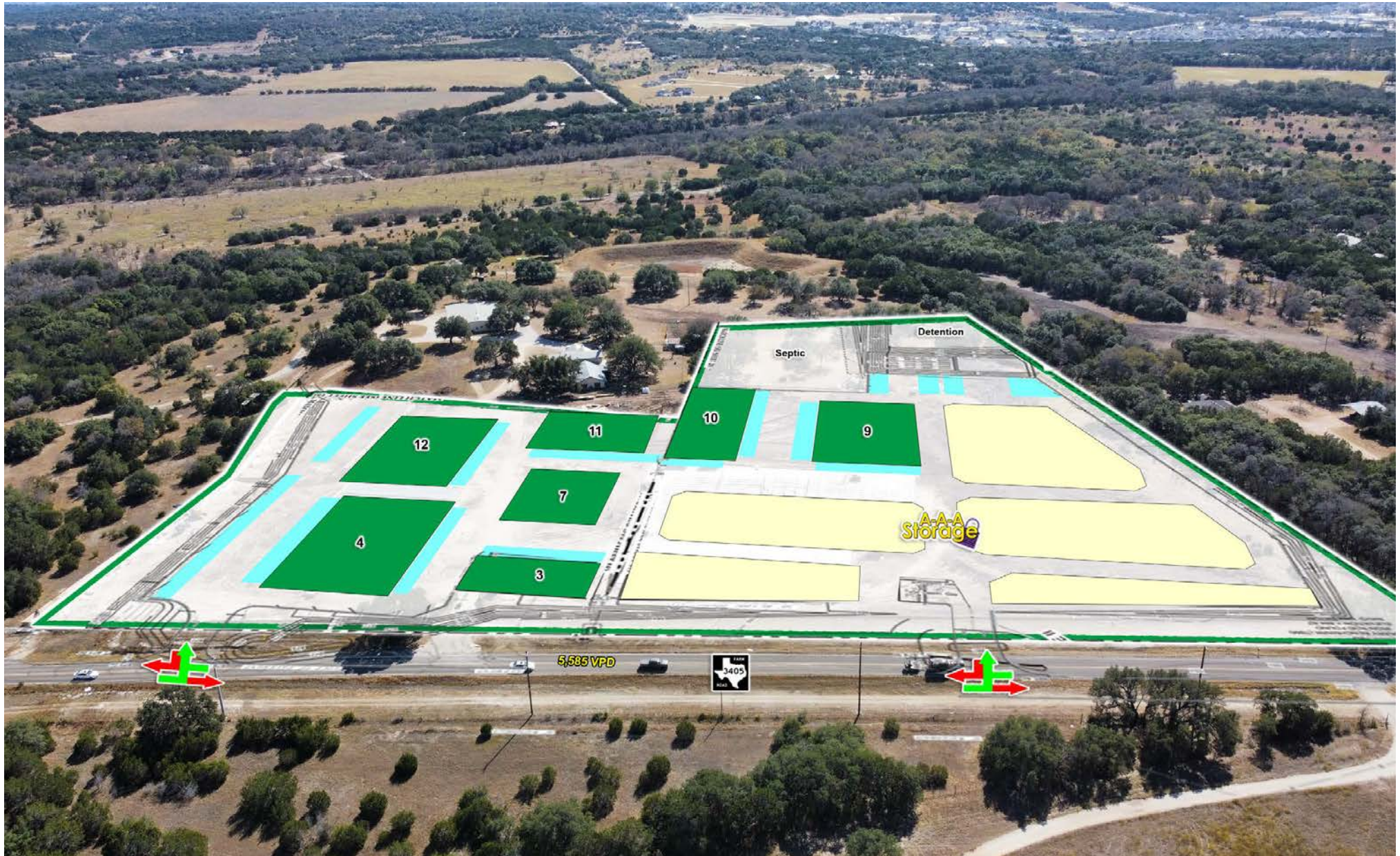
Construction Progression Nov 2024
