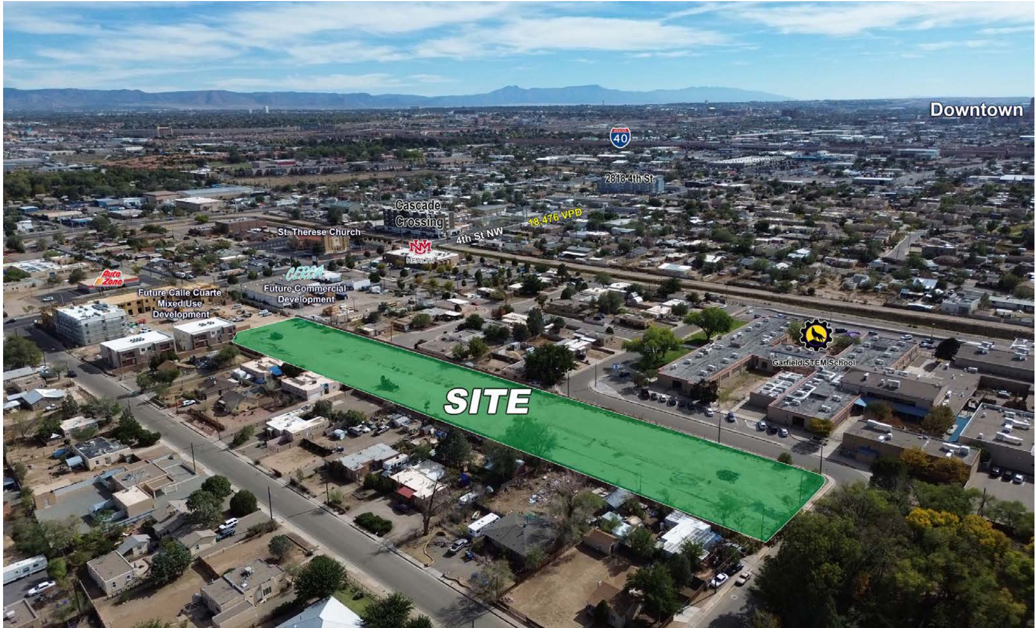
Construction Progress as of October 2024
