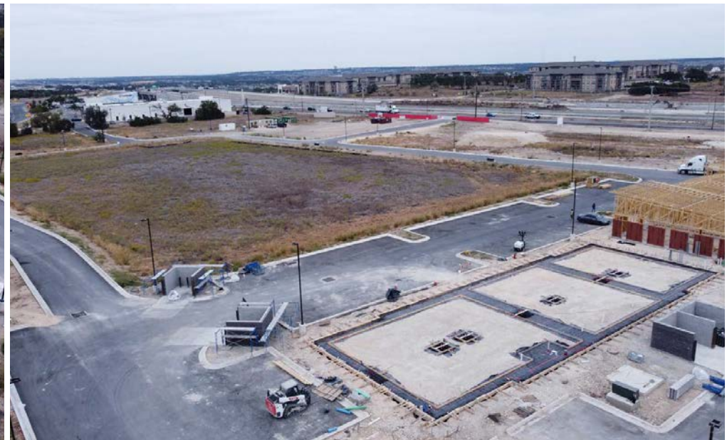
Construction Progress Oct 2024
