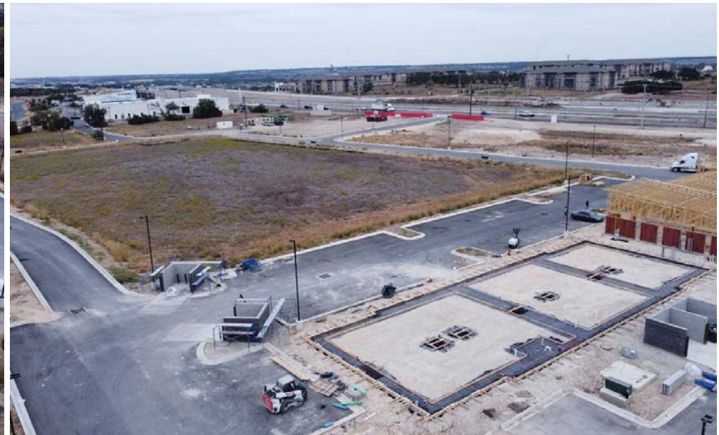
Construction Progress Oct 2024
