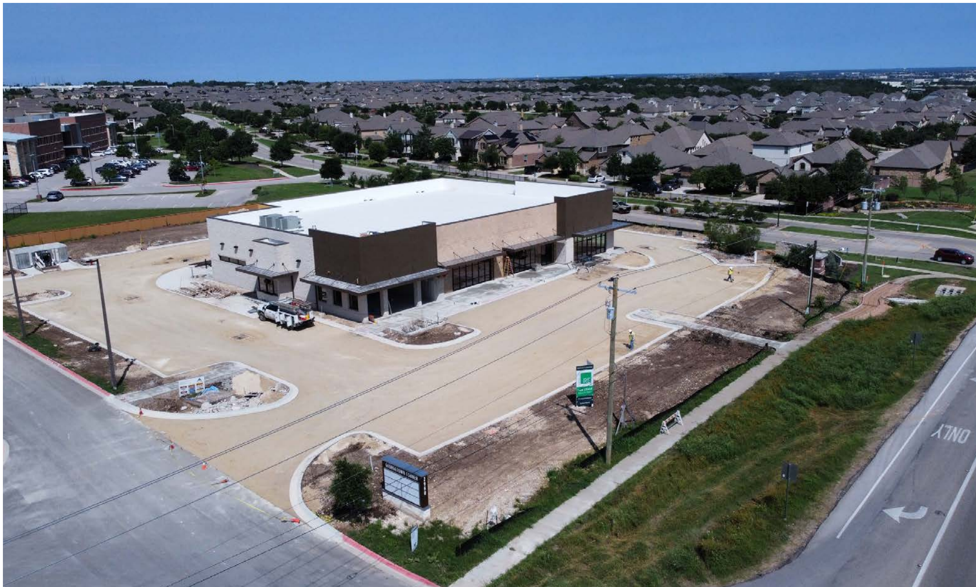
CONSTRUCTION PROGRESS MAY 2024
