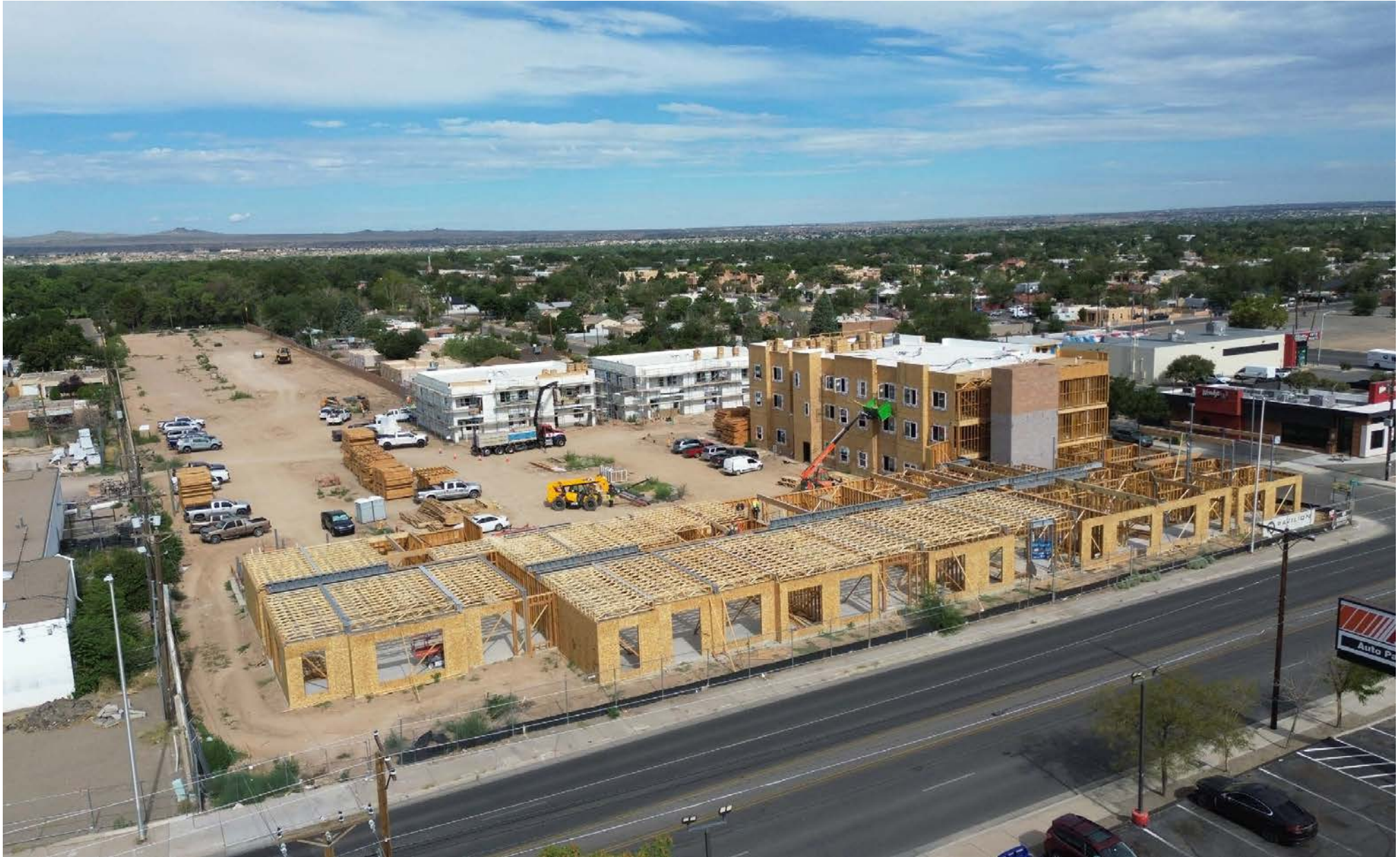
Construction Progress as of August 2024
